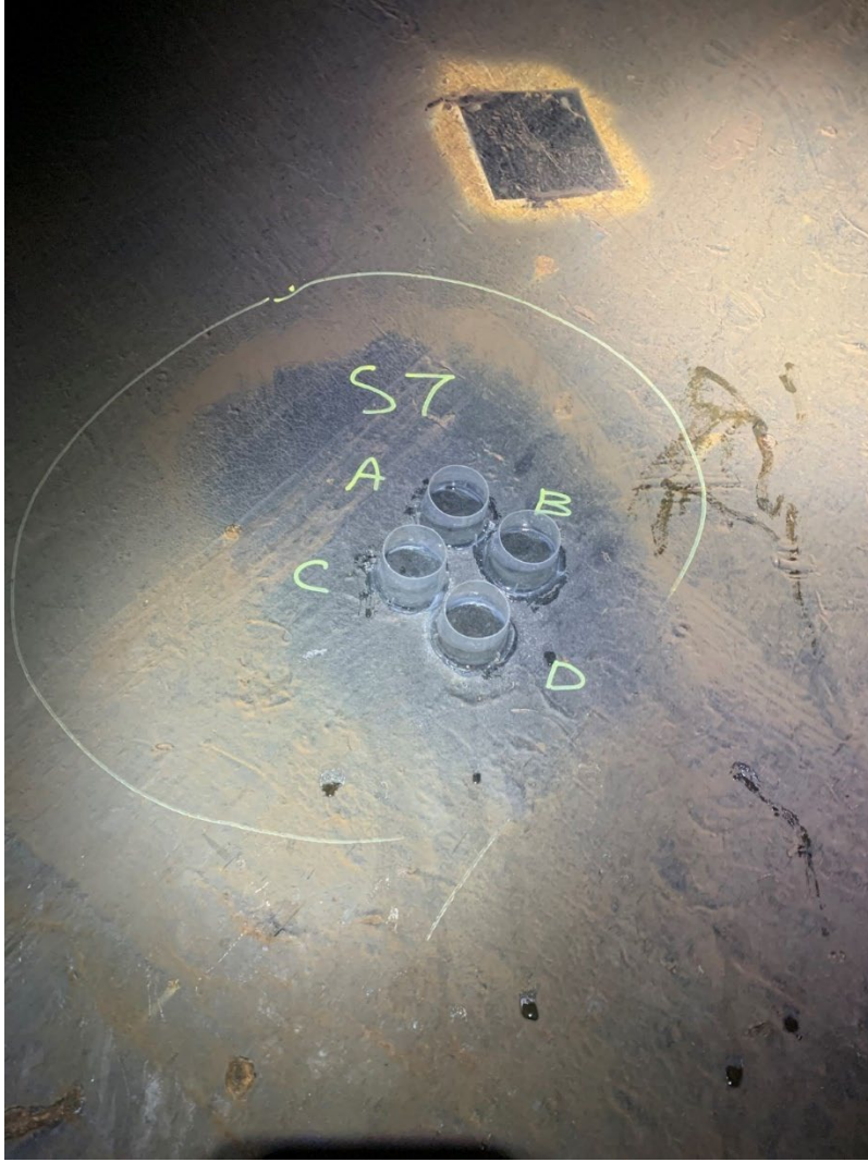
Figure 8. EIS location S7 coal tar CA-50 (System 7)
