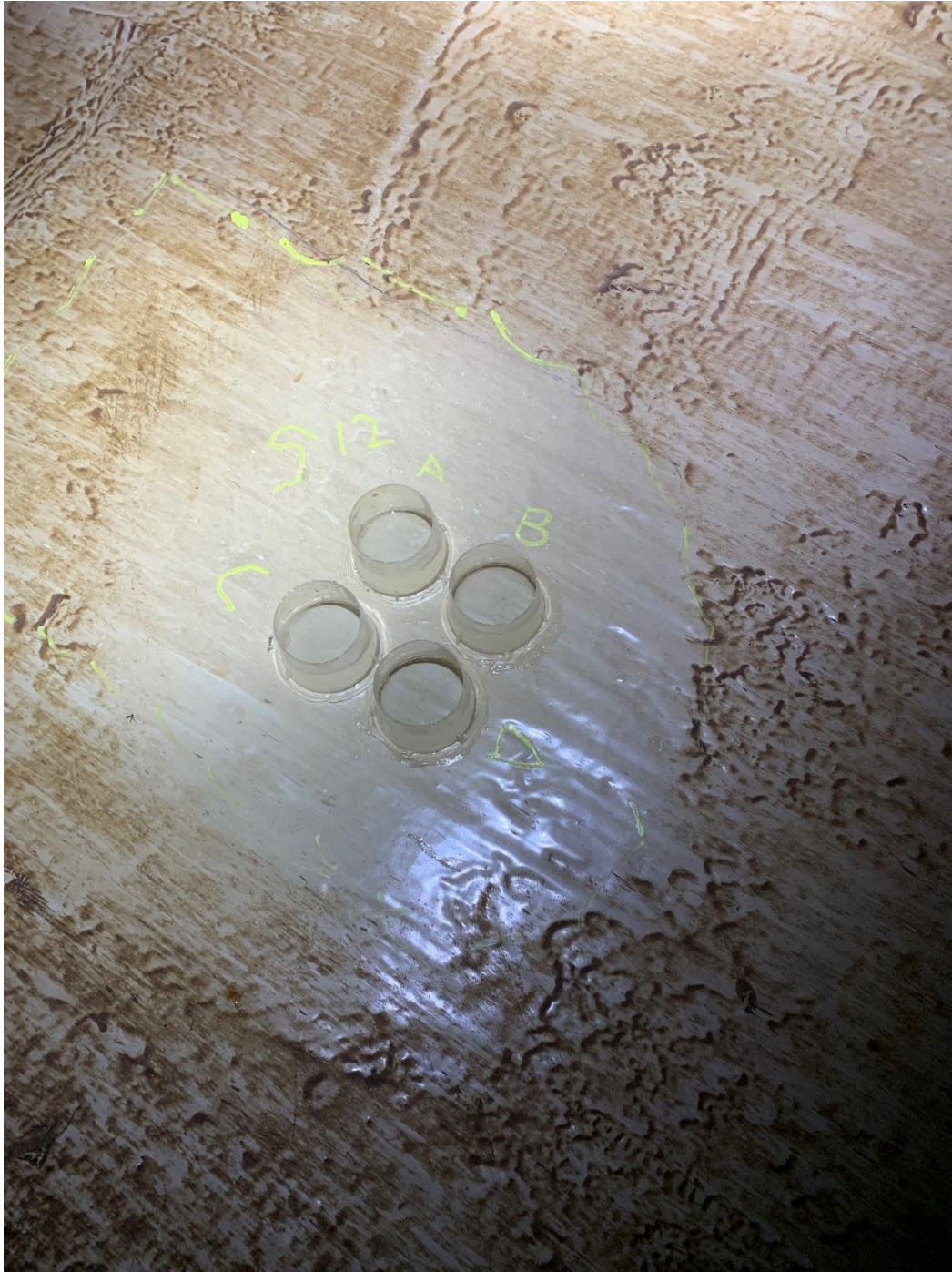
Figure 18. EIS location S12, 100-percent solids epoxy.
