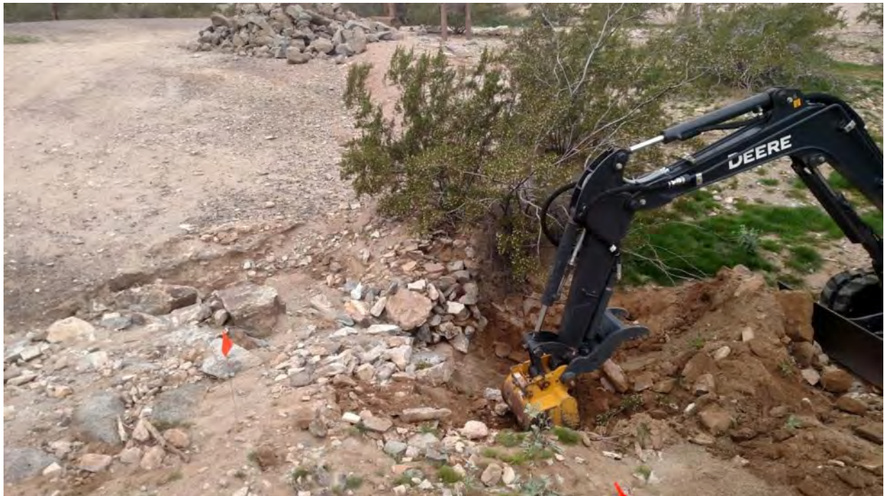
Figure 10. Excavating for Zuni Bowl installation.
