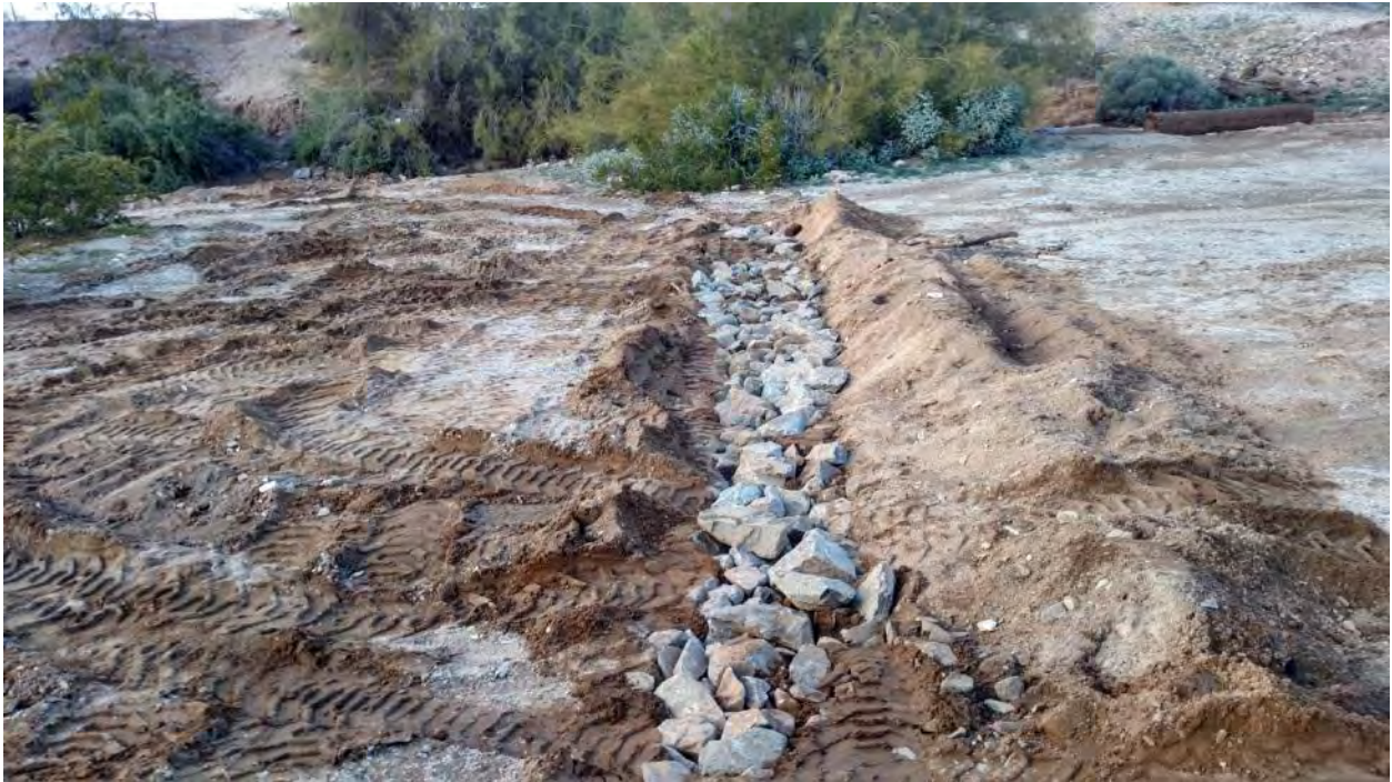
Rock Sill – on floodplain at end of reach, January 2019
