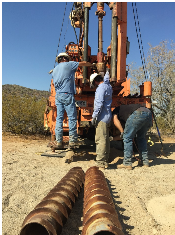
July 7, 2017 Reclamation drill crew Robert Firasek, Willie Nelson, and Jordan Mogdolino installing two monitor wells at the HSP.
