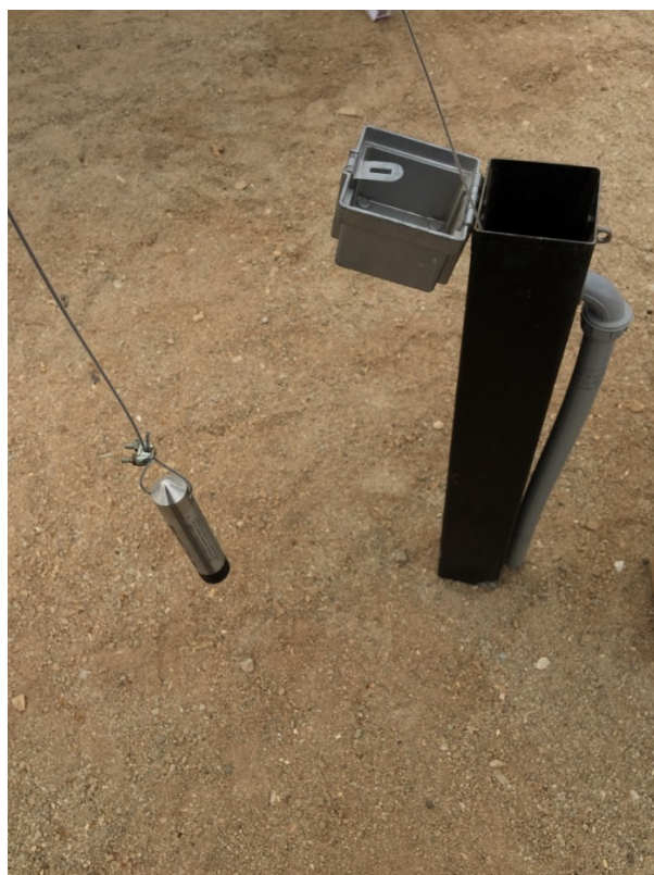
July 7, 2017 HSP-2 Transducer installation in monitor well HSP-2.
