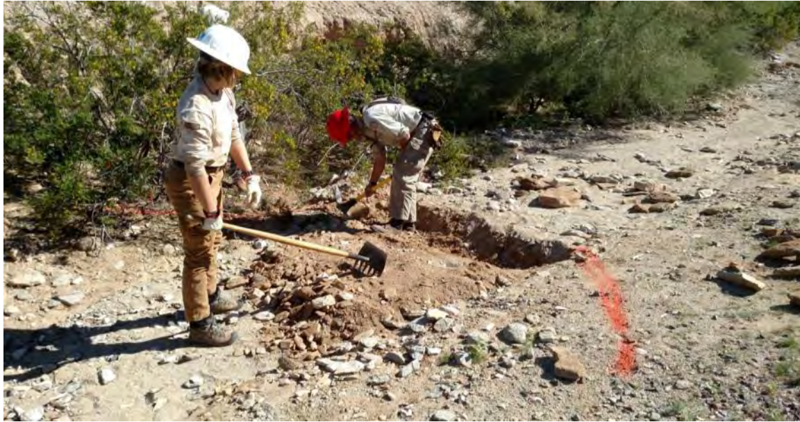
Figure 4. Excavating for structure placement.
