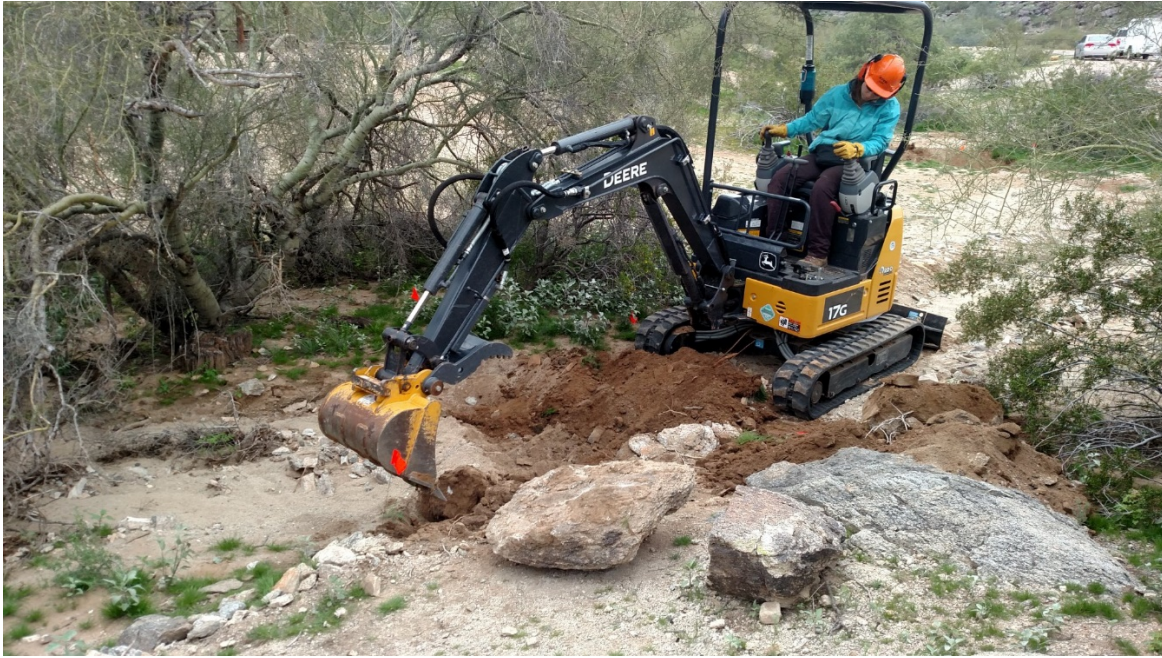
American Conservation Experience (ACE) excavation for Grade Control Structure installation.
