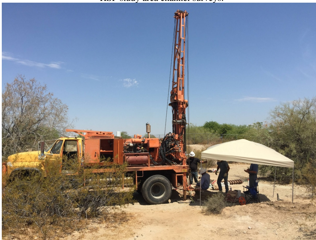
7/7/17 Reclamation drill crew and regional geologist drill and install two wells at the HSP.
