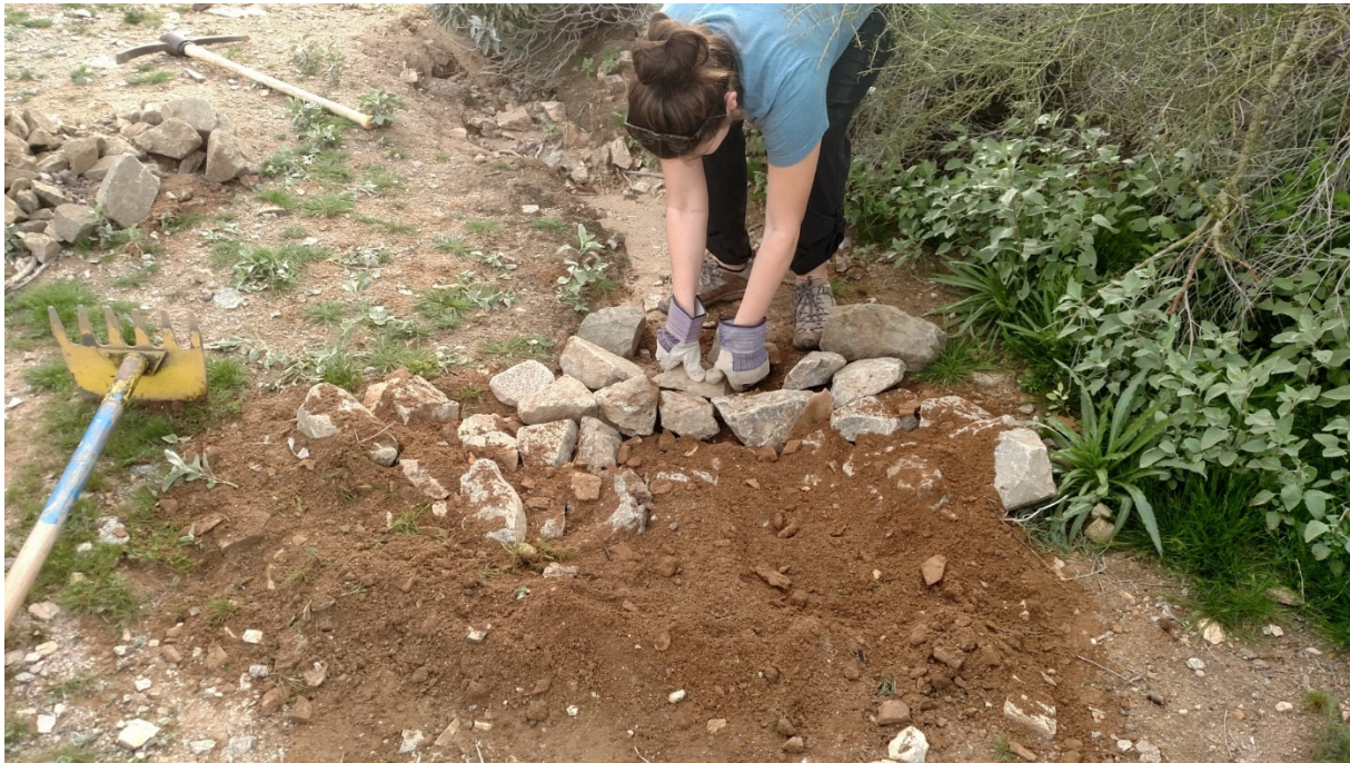
American Conservation Experience (ACE) building Grade Control Structures.
