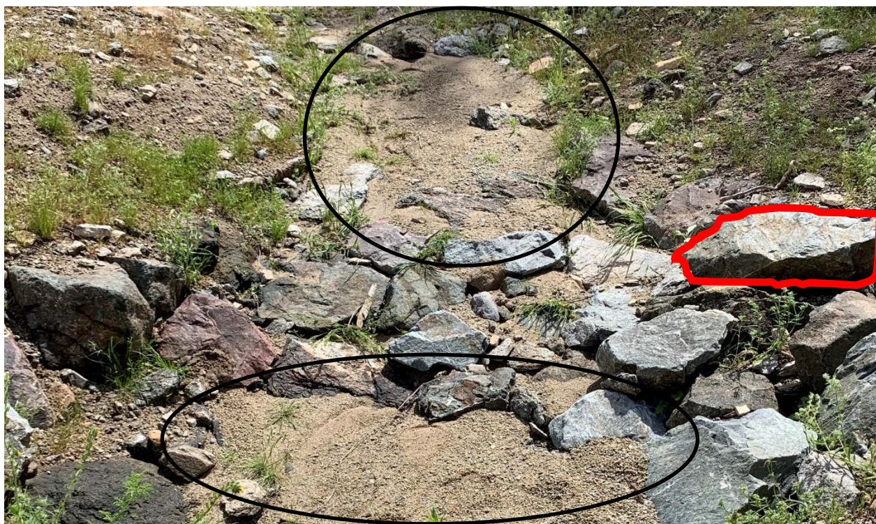
Sedimentation at Grade Control Structure #1 Looking Upstream, March 2020.
