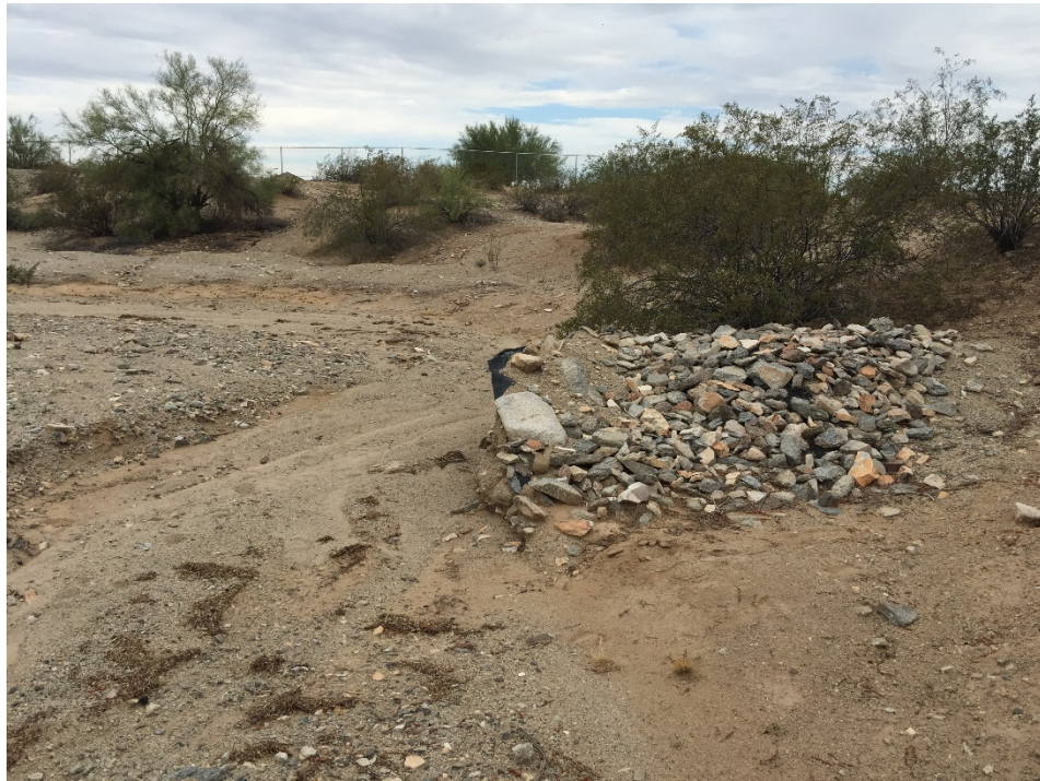
Remnant grade control feature in HSP channel.
