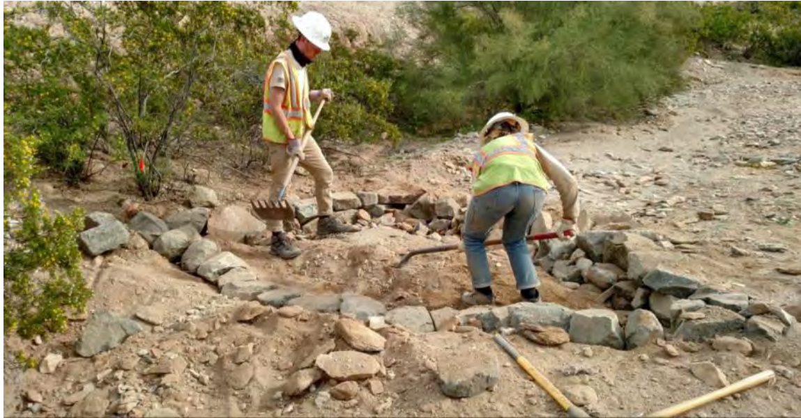
Figure 6. Grade control structure with weir and downstream rocks installed.
