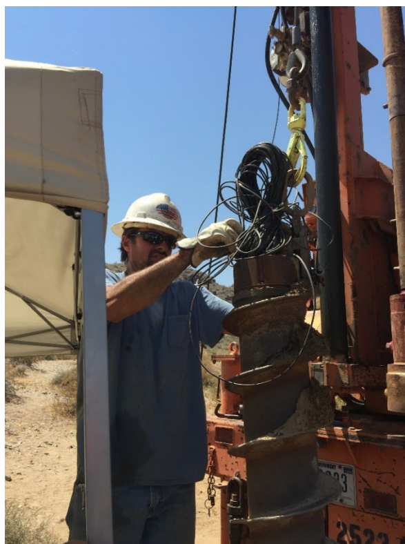
July 7, 2017 Robert Firasek (Reclamation) feeds soil moisture sensor cables into the HSP-2 borehole.
