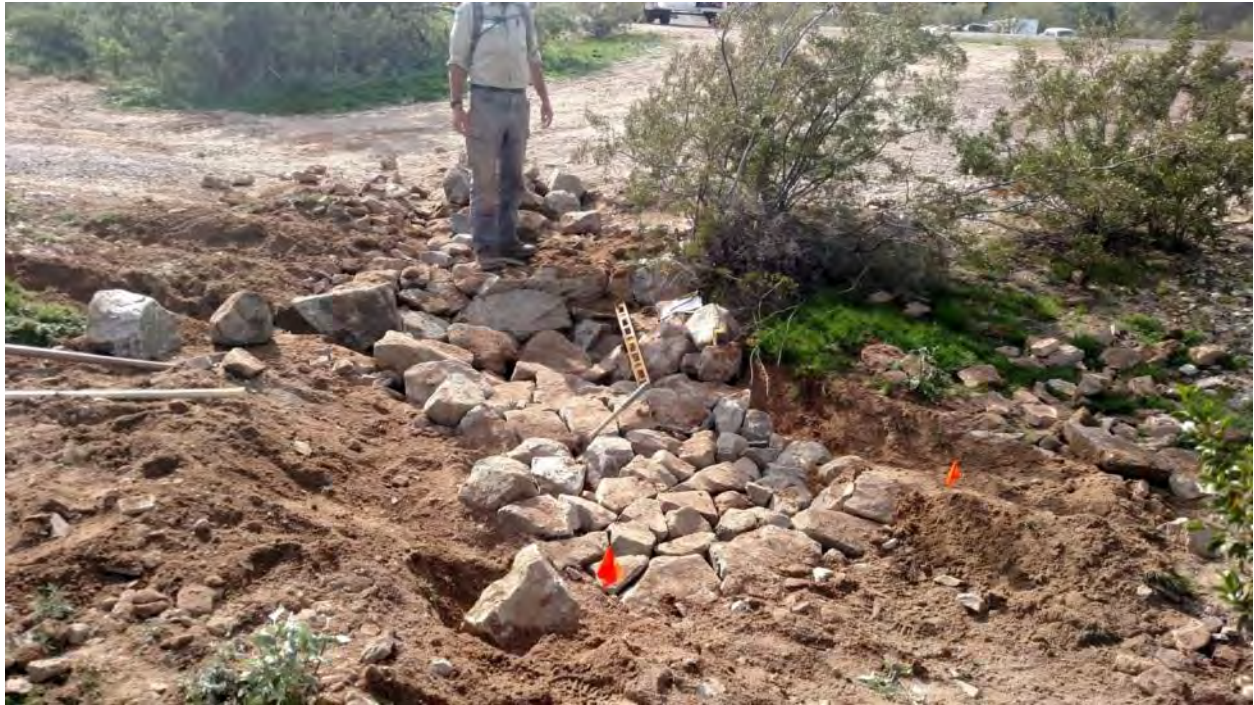
Figure 11. Placing rock into Zuni Bowl
