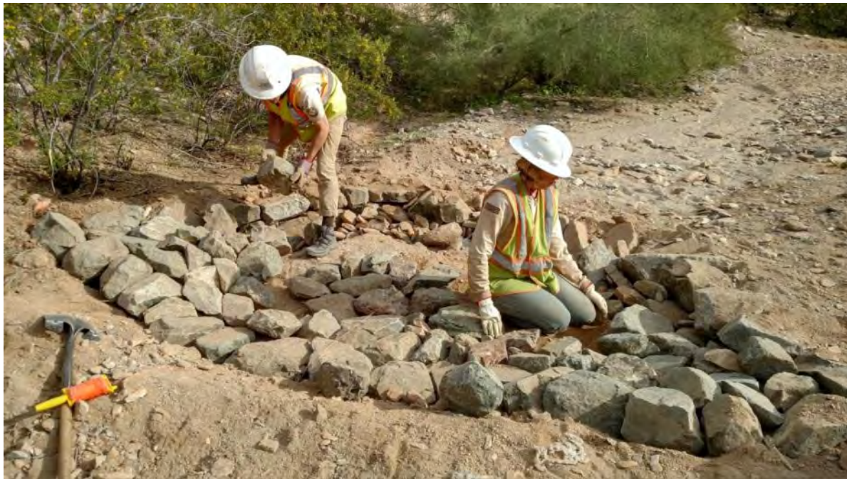
Figure 7. Placing rocks in the interior of the structure.
