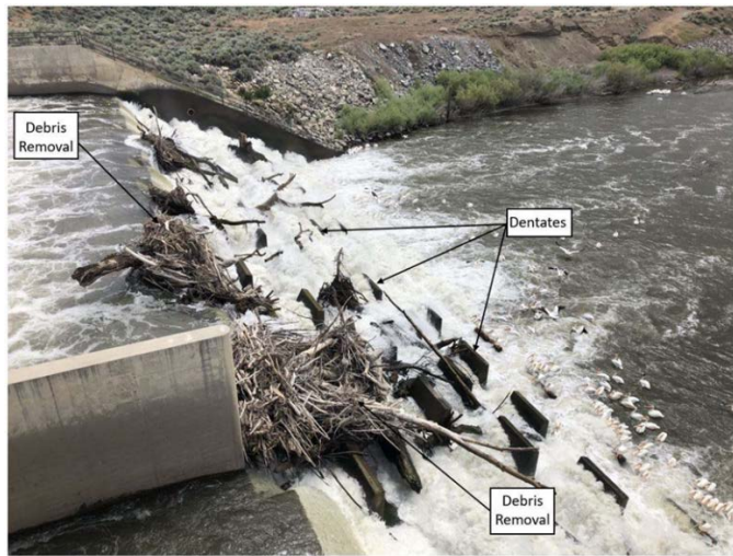
Figure 14. Medium-sized woody debris caught in dentates at drop structure on Marble Bluff Dam, Nevada.
