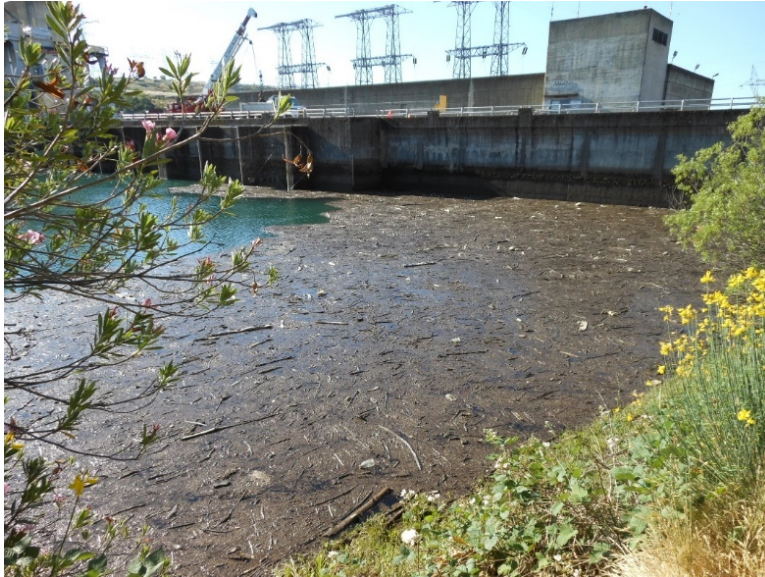
Figure 4. Small- to medium-sized floating woody debris and vegetative debris against Keswick Dam, California.
