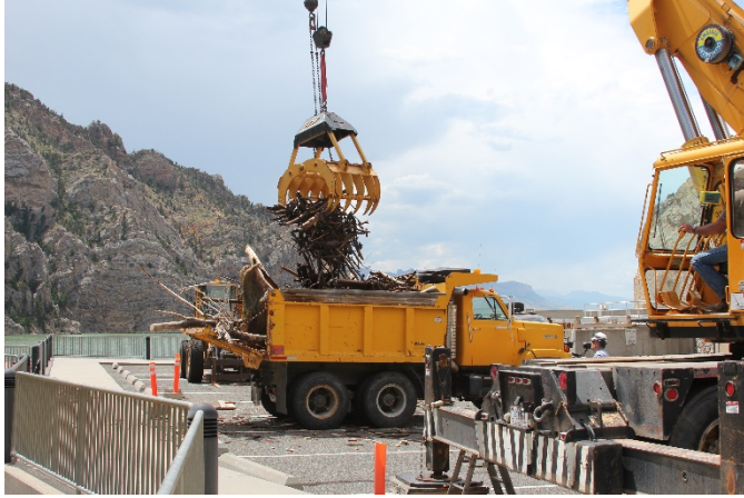
Figure 13. Removed debris at Buffalo Bill Dam, Wyoming, is hauled by truck.
