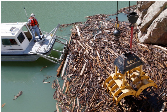
Figure 12. Medium-sized deadfall trees accumulated at Buffalo Bill Dam, Wyoming. Surface debris piled against the face of the dam is removed annually depending on resource availability (typical removal effort is 1 - 2 weeks). A large rake attached to a front end loader is used to remove wood debris on the reservoir bed.
