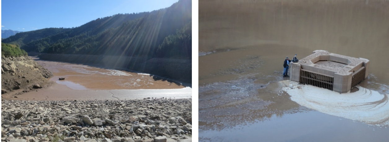
Figure 10. Photograph from Paonia Dam in Colorado showing sediment deposition in the reservoir (left) and at the intake structure (right). Small debris is not too big to fit through the trashrack openings if oriented lengthwise, but debris that impinges on the trashrack allows sediment to back up behind it.
