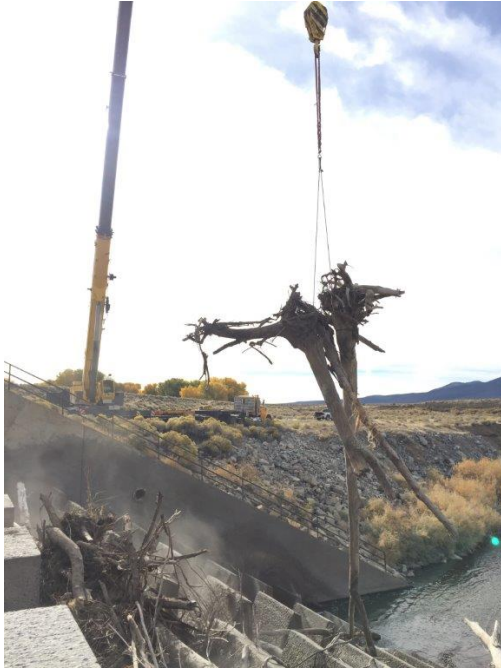
Figure 15. Removal of deadfall by crane at Marble Bluff Dam, Nevada.
