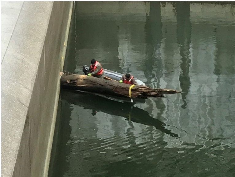
Figure 5. Manual removal of large log from Morrow Point Dam, Colorado.
