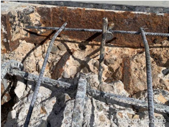
Figure A-4.—This structure has documented issues with ASR. Left: deteriorated concrete due to ASR. Right: Old concrete removed from around reinforcing steel prior to repair.
