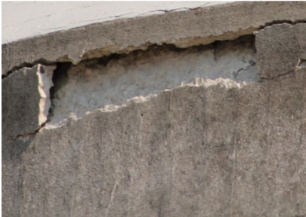
Figure A-4.—This structure has documented issues with ASR. Left: deteriorated concrete due to ASR. Right: Old concrete removed from around reinforcing steel prior to repair.
