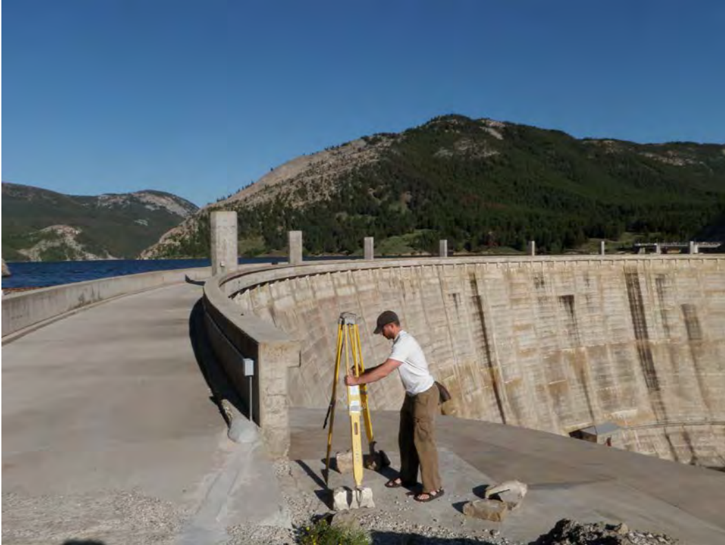
Figure 3 - GPS control point, Set 2, located in the top of the dam near the right abutment.
