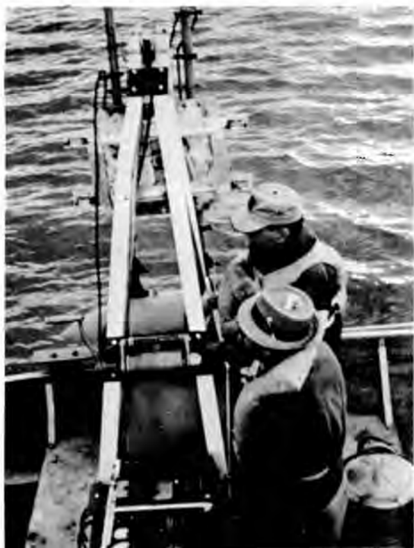
Figure 4. Sonic depth recording equipment. Transducer is out of water. Photo P258-D-57761
