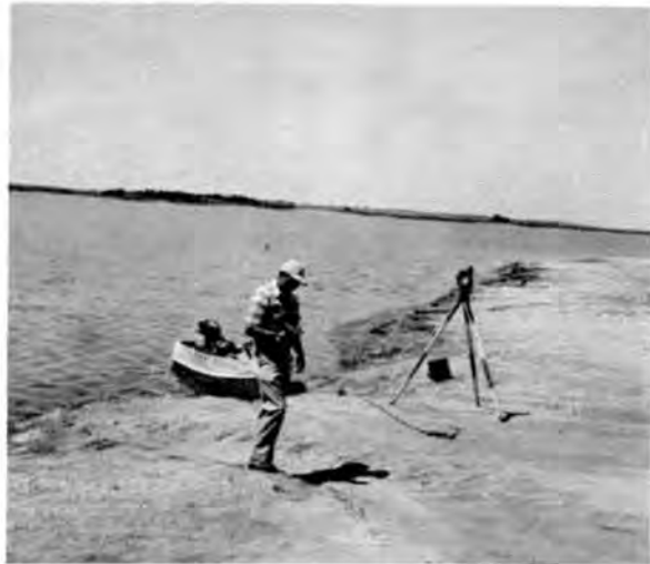
Figure 7. Transit set up on range point in line with R7L at water's edge. During the sounding operation the man on shore keeps the boat on line through the transit. Radios are used for communication between the transit man and the boat operator. Photo P258-D-57711
