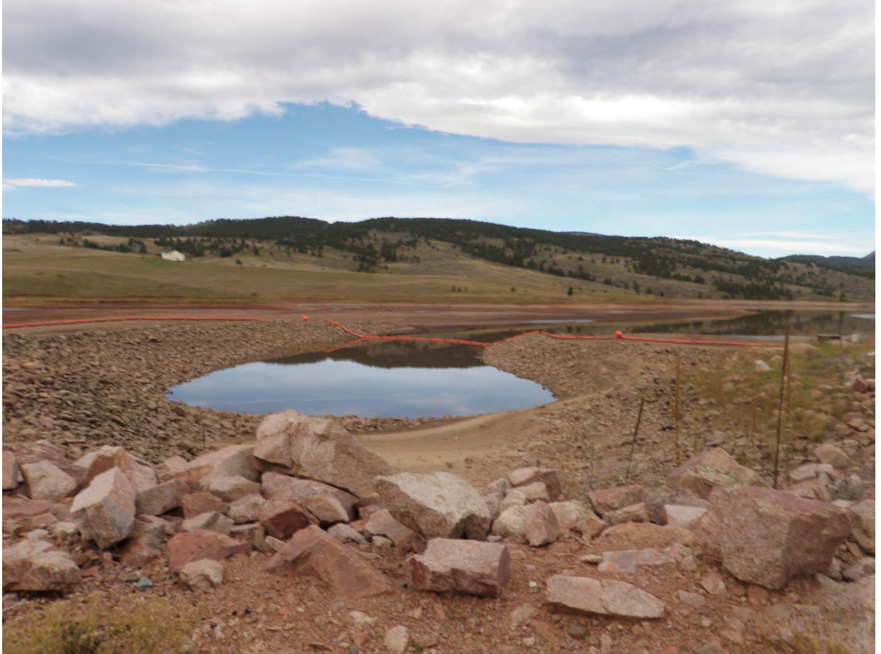
Figure 2 - Intake to Bald Mountain Pressure Tunnel to the Flatiron Powerplant with reservoir drawdown about 20 feet below normal full pool elevation 6,580.
