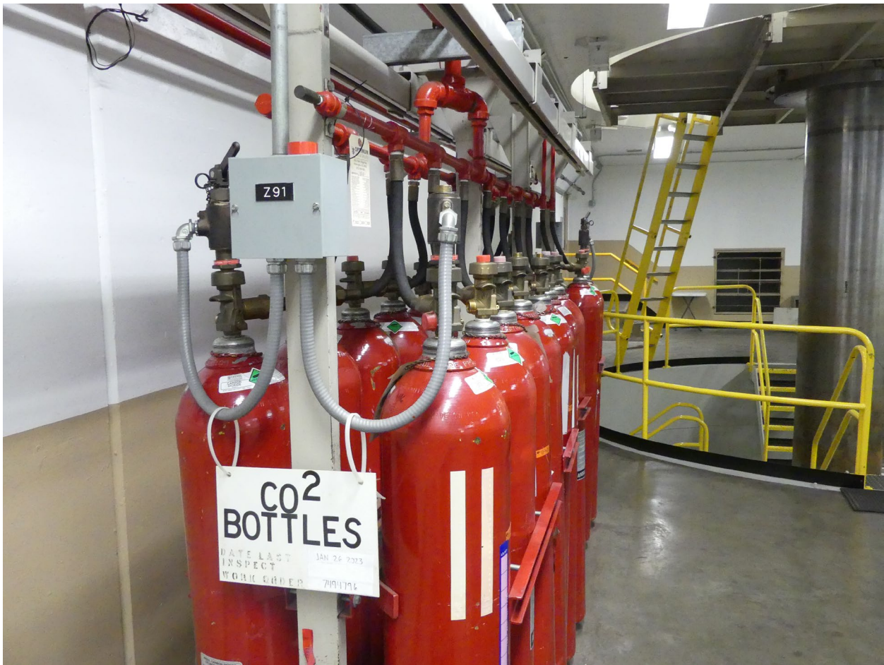
Figure 3. —Typical high-pressure CO 2 system commonly found in Reclamation. Multiple CO 2 cylinders are connected by hoses to a common manifold.
