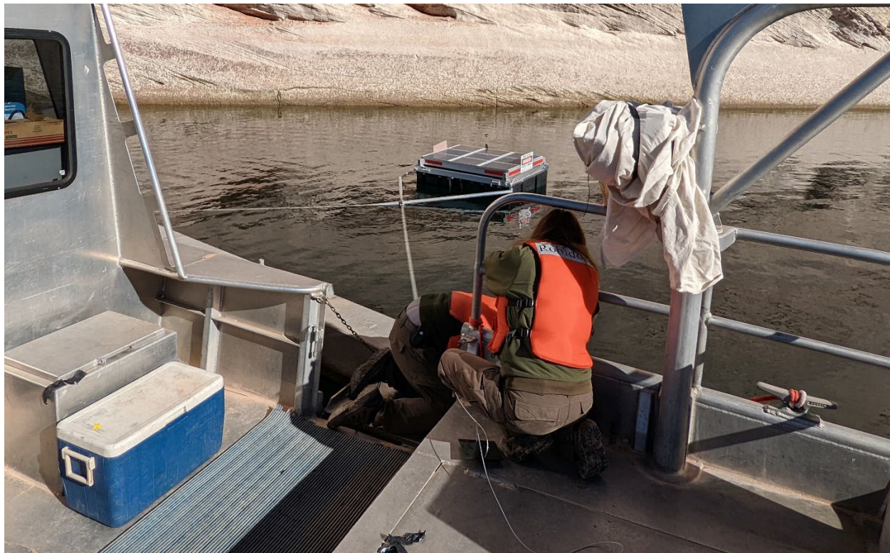
Figure 2. Installation of the ultrasound solar raft on the east side of the GCB Site.
