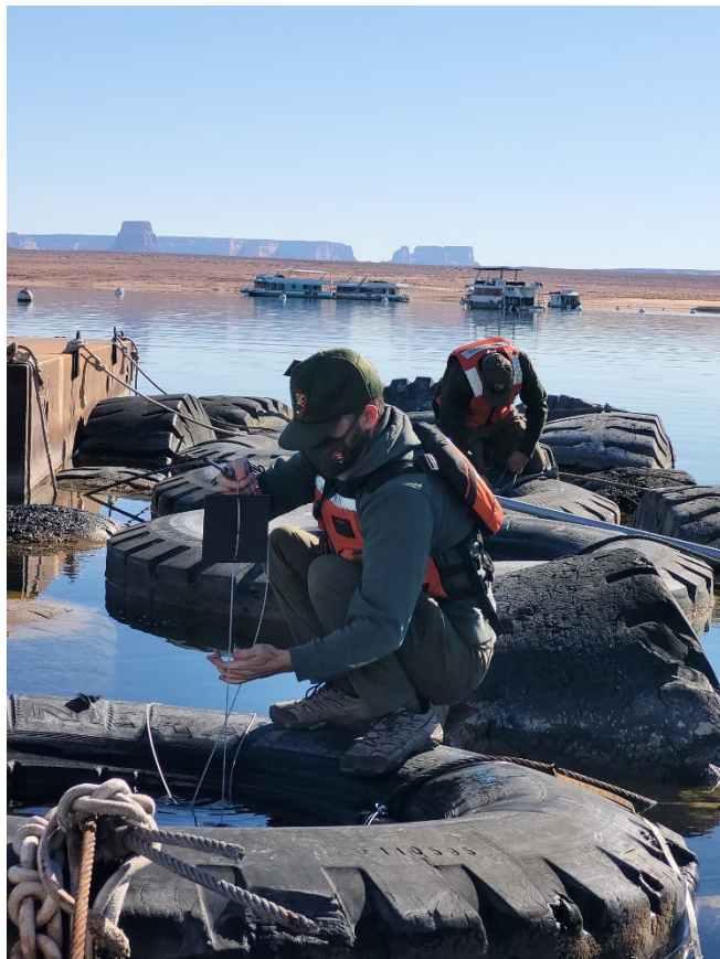
Figure 5. Installation of settlement plates by NPS staff at the SLB site.
