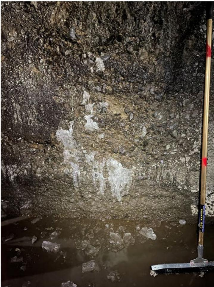
Figure 32.—Photos of tunnel conditions showing uneven concrete surface (top) and icy walls (bottom) due to the deterioration of the concrete.
