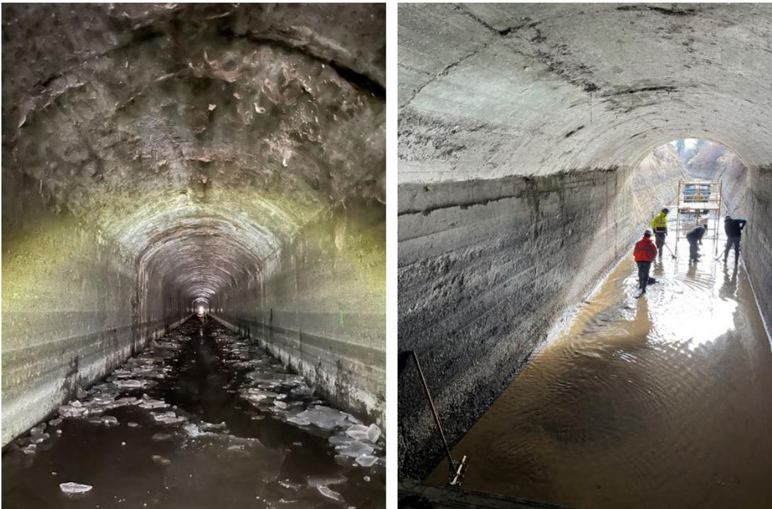
Figure 34.—Photos of tunnel conditions showing cobwebs across ceiling with broken up icy floor (left) and deepening standing water (right).
