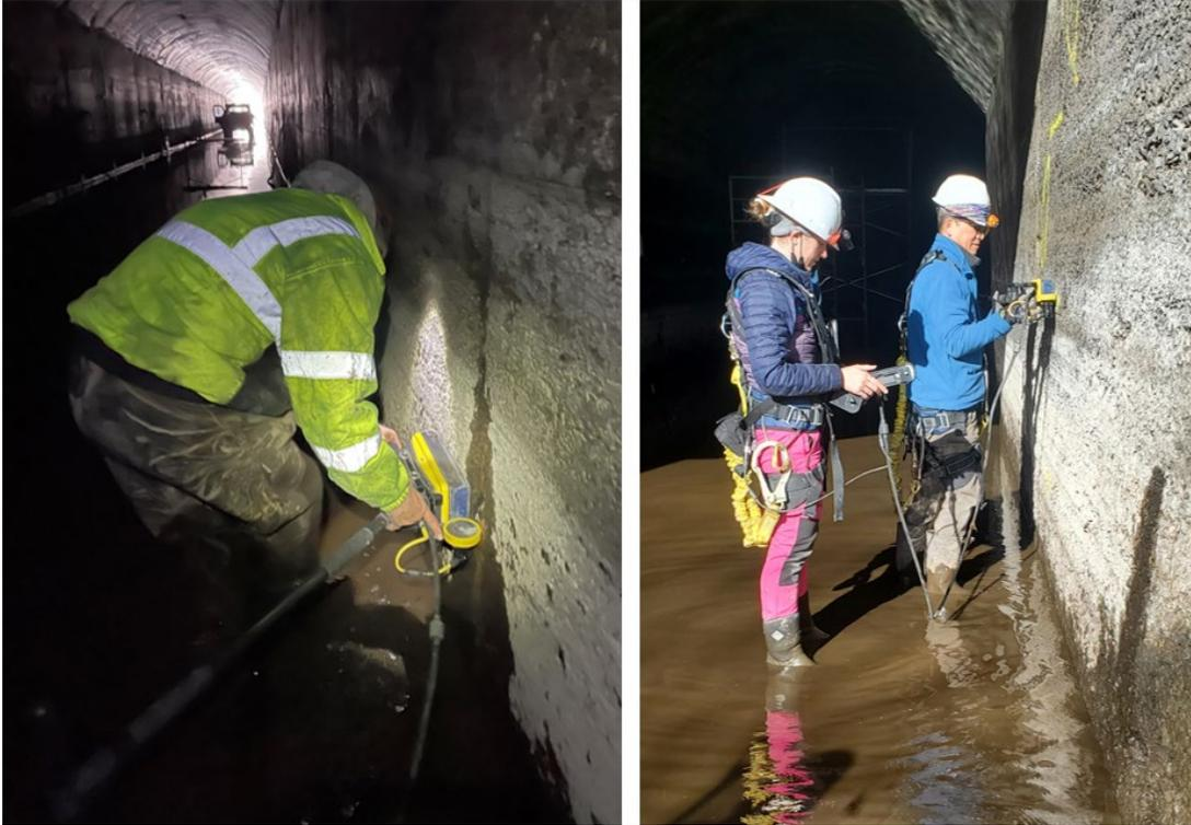
Figure 33.—Photos of Reclamation personnel performing GPR surveys on the tunnel walls.
