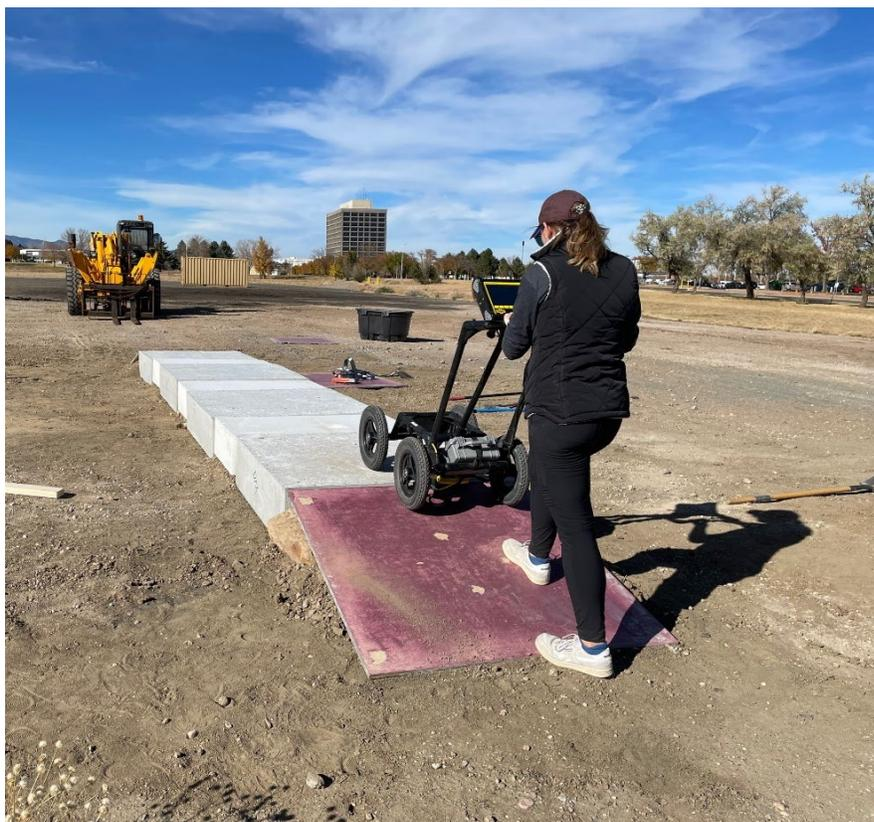
Figure 16.—Photo of ramp construction on each end of survey area to aid GPR surveying.
