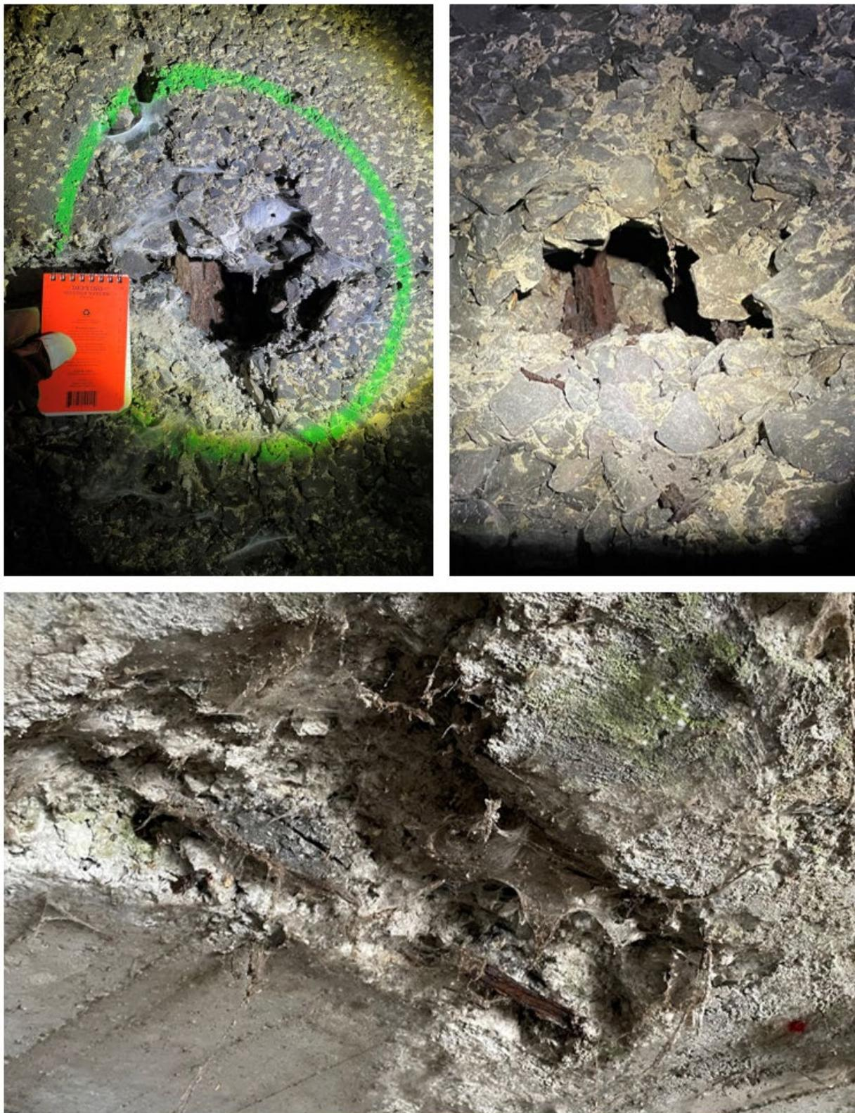
Figure 31.—Photos of exposed timber reinforcement and varying degrees of concrete deterioration observed in A Canal Tunnel during data collection.
