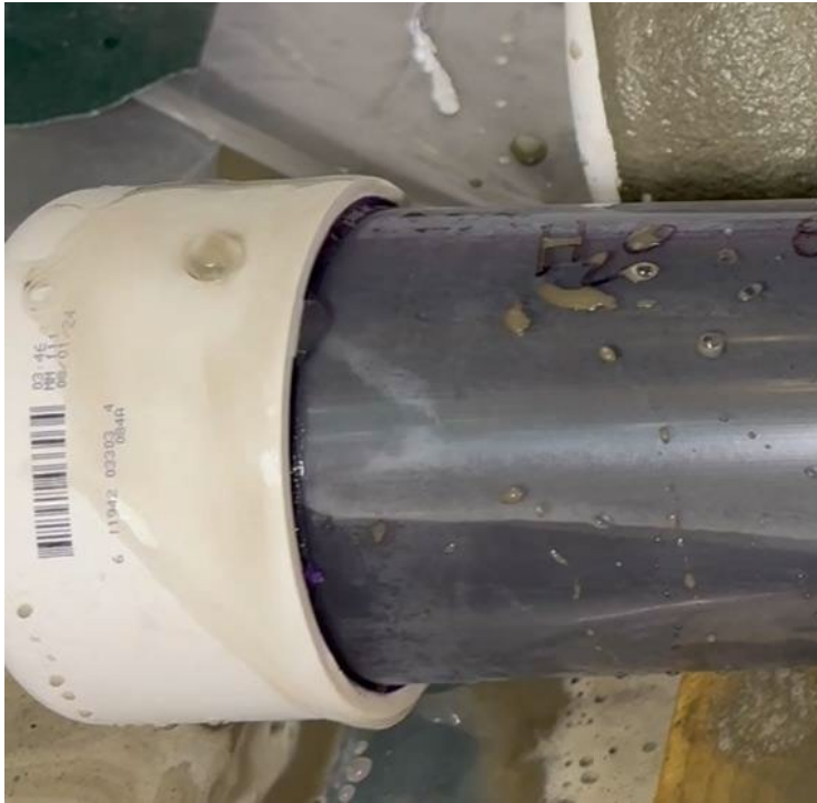
Photograph 23.—Clean water discharging from vent hole during placement of PLDCC.
