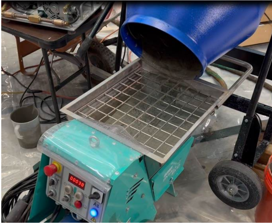
Photograph 3.—PLDCC transferred from drum mixer to grout pump.
