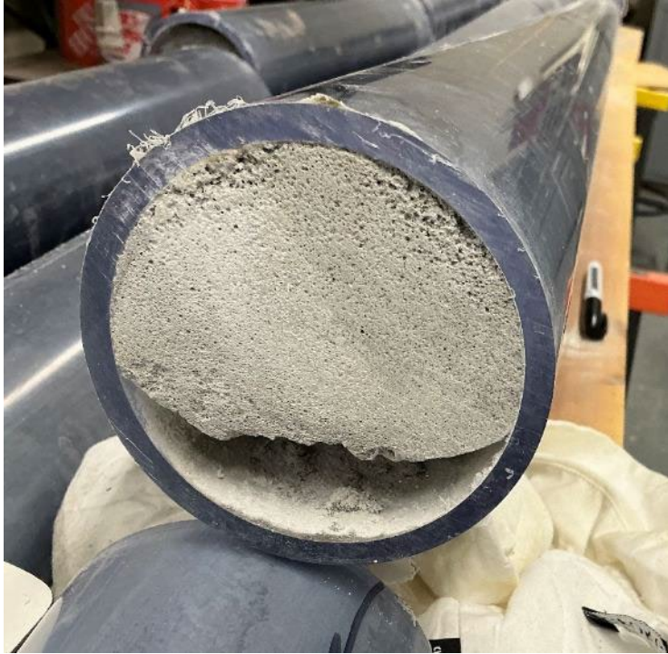
Photograph 24.—PLDCC specimen from 8-foot horizontal-water, with water-filled void at bottom pipe at vent end.
