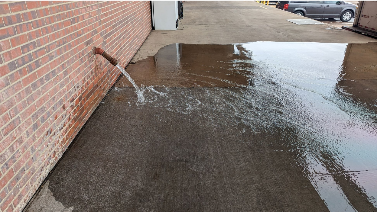
Figure 20.—Photo of the water release outfall onto an exterior loading dock, taken during initial testing of Nb-IoT loggers at the GSA facilities Building 810 warehouse.
